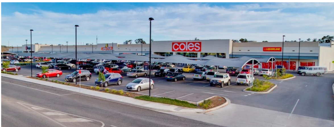
Figure 1. Broken Hill Village, Broken Hill, NSW
