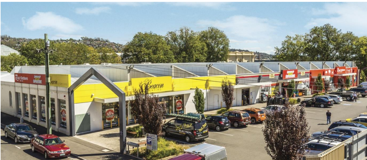
Figure 1. Launceston Homemaker Centre from William Street
